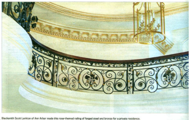
Blacksmith Scott Larkston of Ann Arbor made this rose-themed railing of forged steel and bronze for a private residence.
