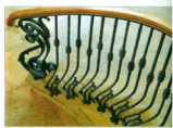
Wrought iron adds weight and sophistication to this staircase's banister complements both wood and stone.
